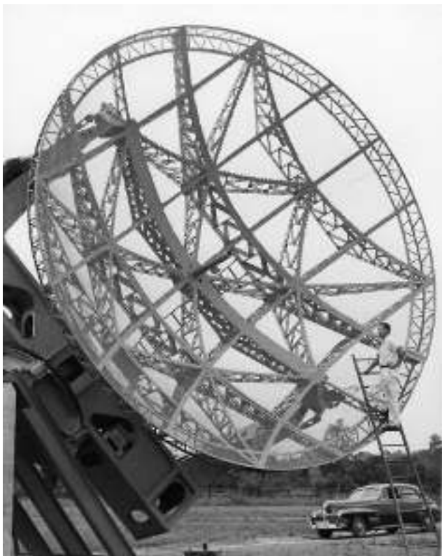
Antenna of a Würzburg radar
